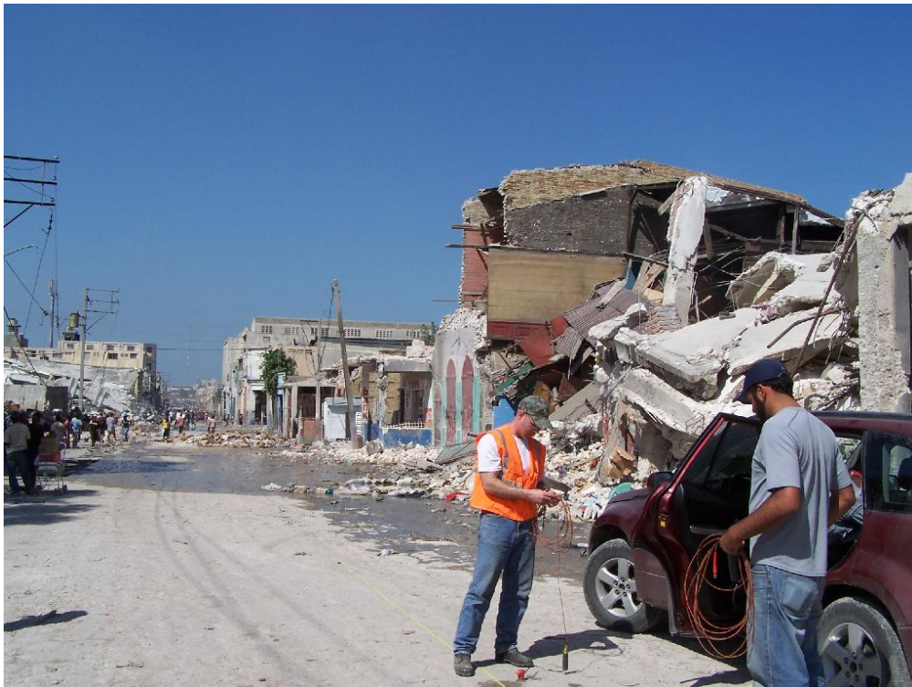
Figure 5.8 Typical types of structures and damage found within the heavily damaged zone near SASW 8 (N18.550210°, W -72.339638°).
